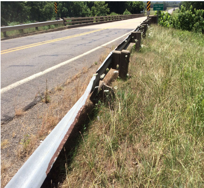
PHOTO 1 Description Northeast bridge rail damage.
