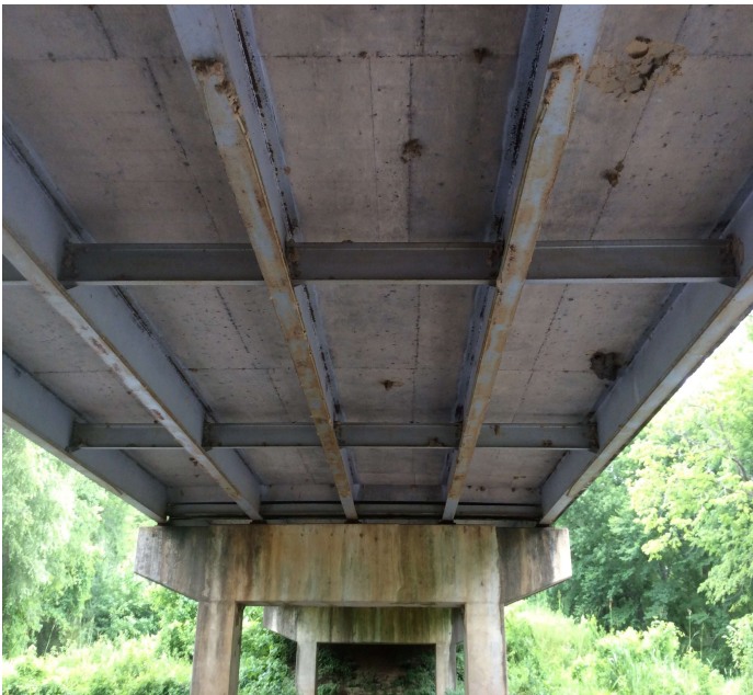
PHOTO 1 Description Typical undersurface of the deck.
