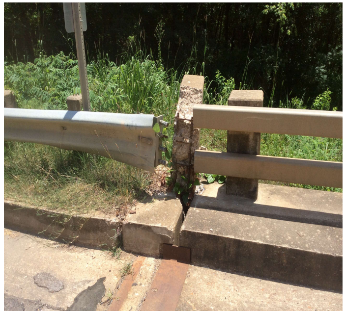
PHOTO 2 Description Southeast bridge rail damage.
