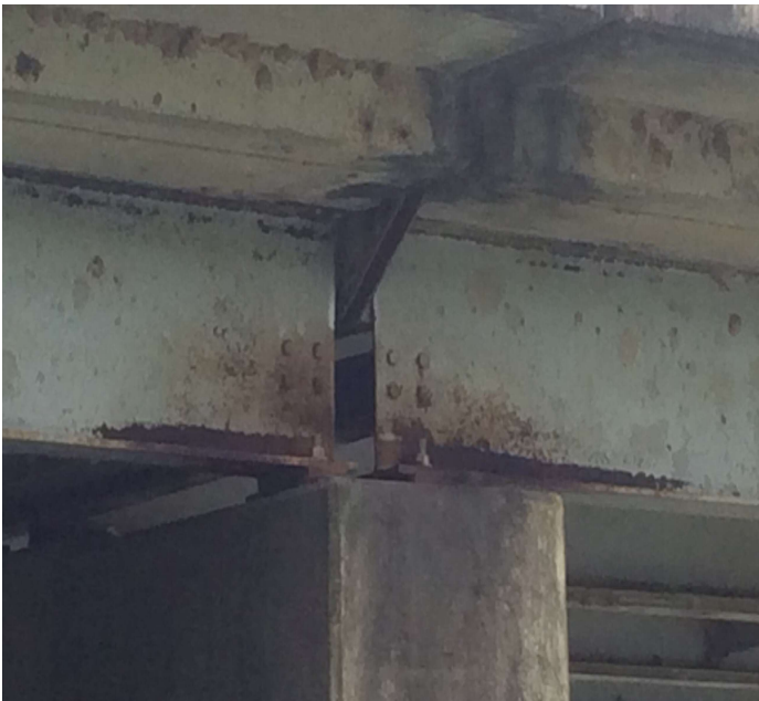
PHOTO 1 Description Active corrosion at the beam ends. No visible cracks in the beams.
