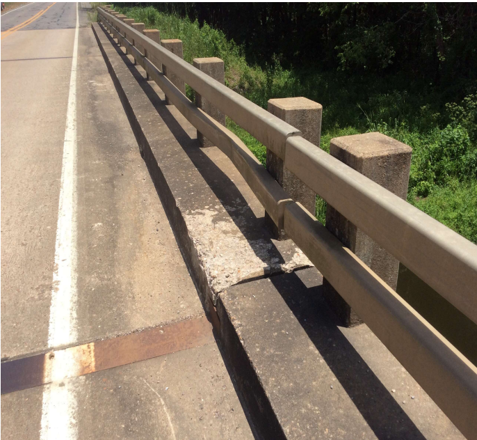
PHOTO 4 Description Span # 4 RT bridge rail damage.
