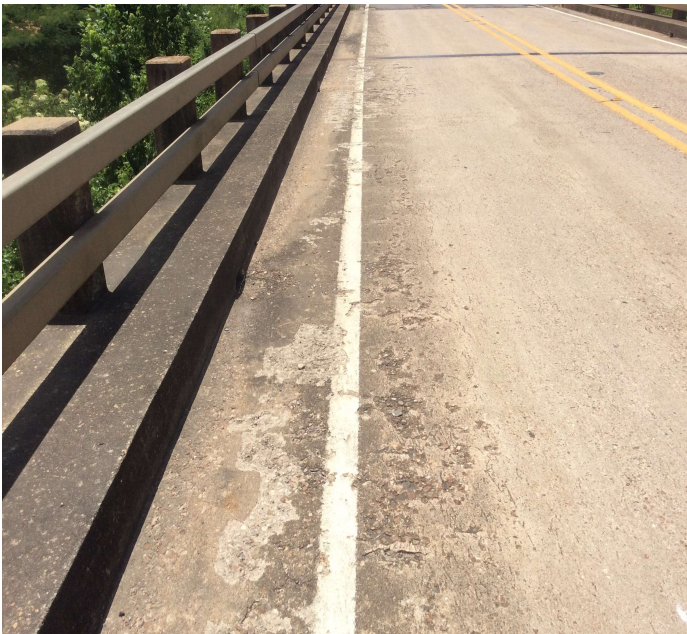
PHOTO 1 Description Concrete delamination in the gutters.
