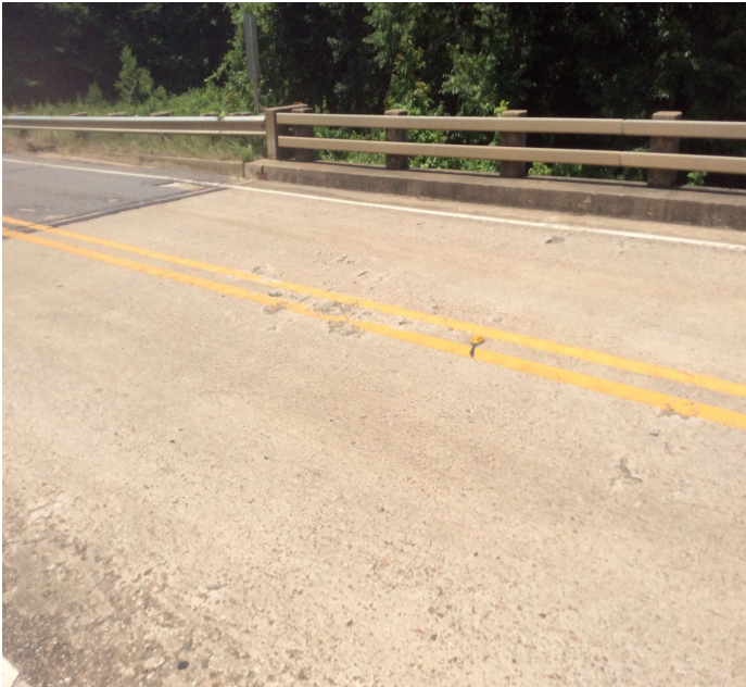
PHOTO 1 Description Span # 1 concrete deterioration.
